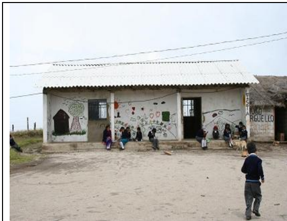
Old structure in Tupac Yupanqui's School.
