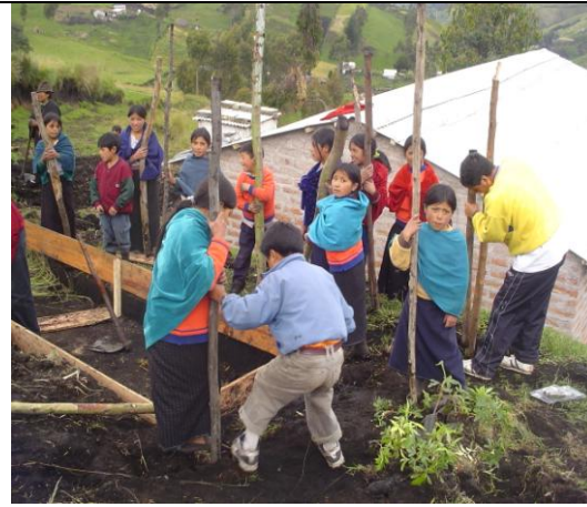
Everybody helping build the fence in Chacabamba Cagrin, 6 de Marzo School
