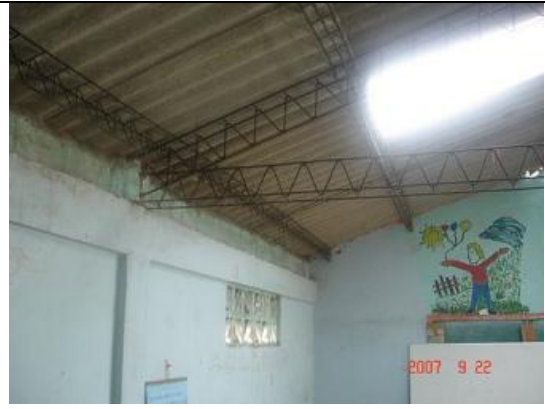
Inside the repaired classroom. Convalecencia School.
