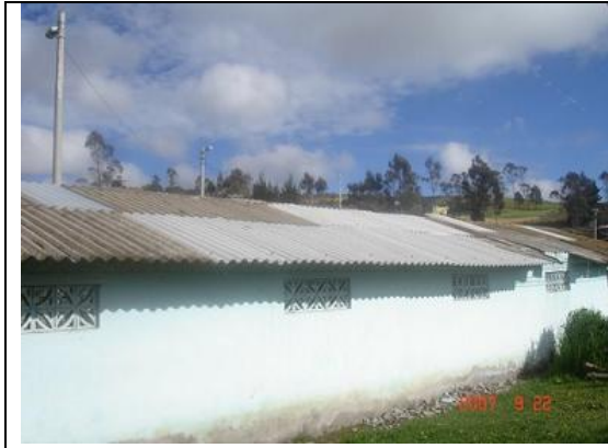
Convalecencia School after ceiling's repair.
